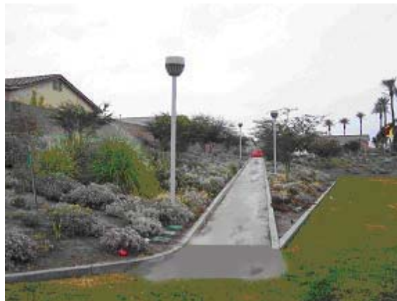
ADA Ramp with Landing and Lighting
