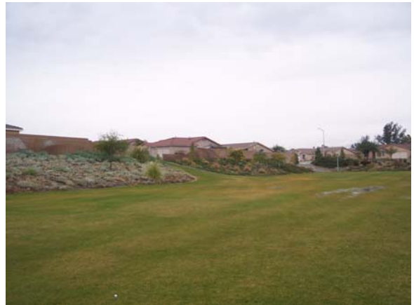
Retention Basin Bottom with Grass
