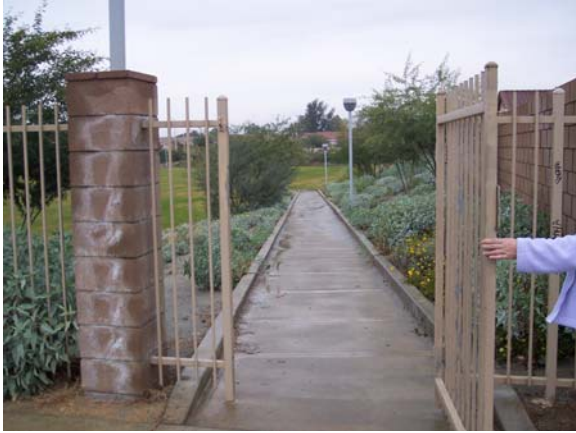
Lockable Personnel Access Gate with ADA Ramp
