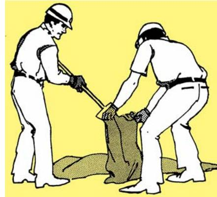
For large-scale operations, filling sandbags can be expedited by using bag holding racks, metal funnels, and power loading equipment. However, the special equipment required is not always available during an emergency. Bags should not be filled more than half full or less than one-third their capacity.
