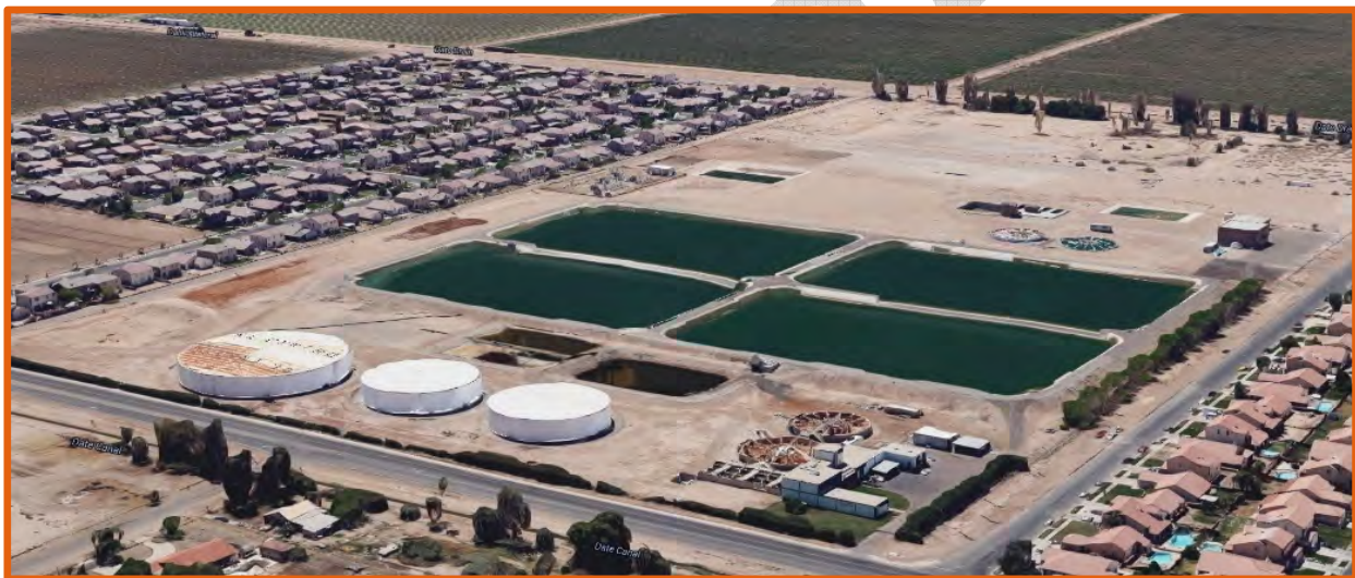
Photo 3-1: El Centro Water Treatment Plant
