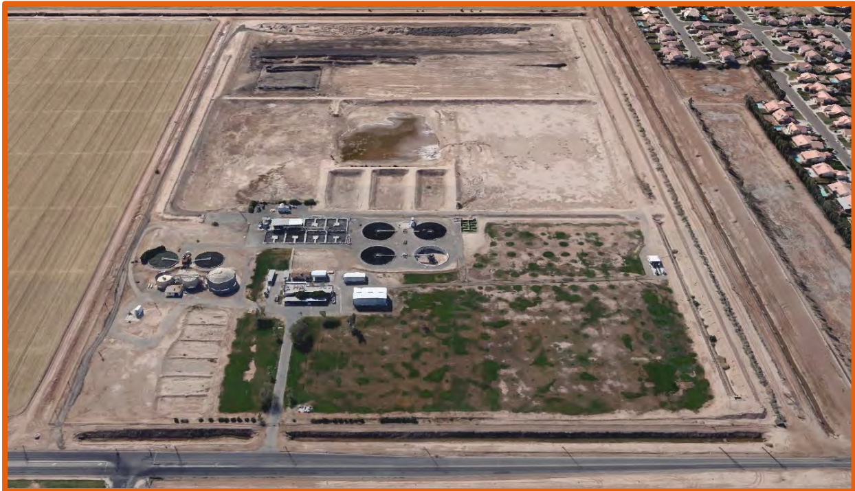
Photo 6-1: El Centro Wastewater Treatment Plant
