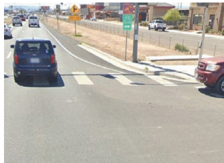
Photo 3: Existing crossing with missing sidewalk
