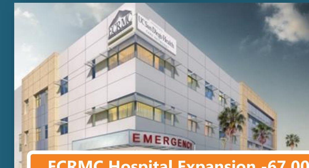
ECRMC Hospital Expansion -67,000 SF
