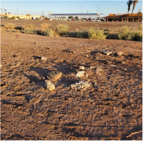
14. Concrete debris on north portion.
