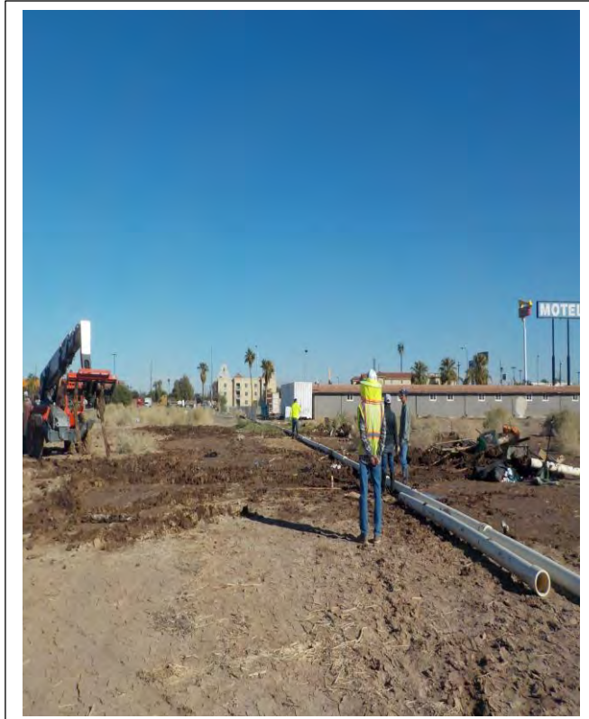
1. Site looking north; water pipe to commercial construction to south
