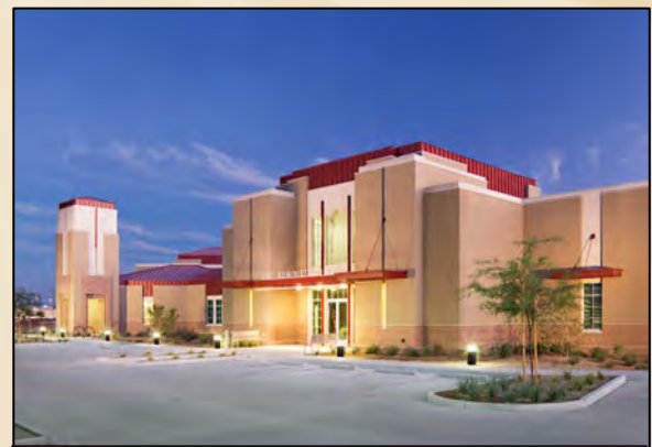
Fire Station No. 3, located at the southwest corner of Waterman Avenue and Bradshaw Avenue.
